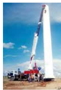
Stand Pipe DN 1800mm
