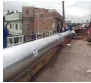
Travessia DN 600mm
