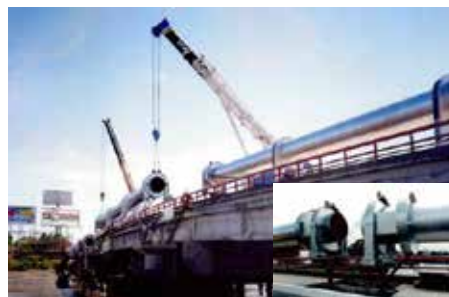
Travessia DN 1200mm
