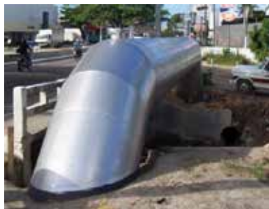
Travessia DN 1200mm
