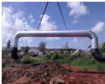
Travessia DN 700mm
